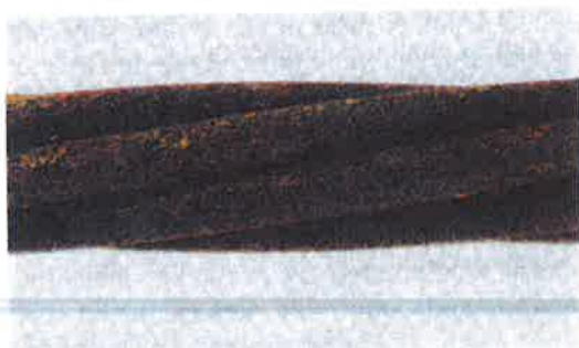
Photo 7. Strand surface before cleaning
