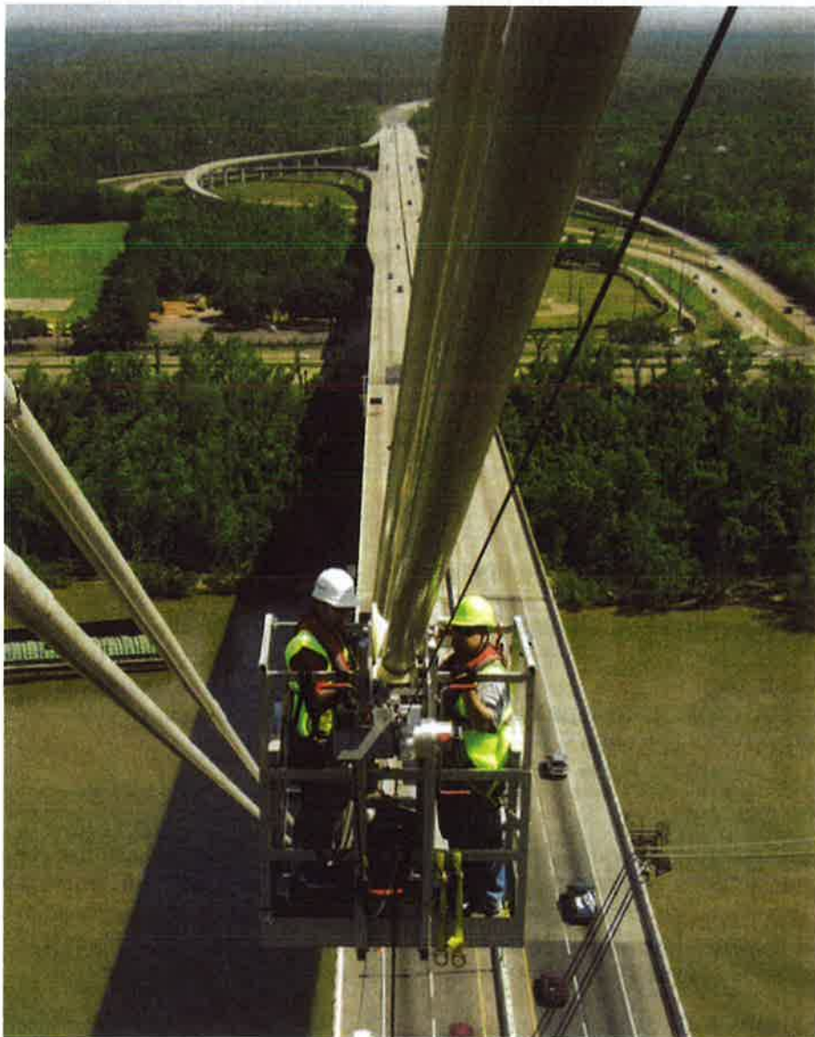
Fig. C7.1—Inspection trolley in use on the Hale Boggs Bridge near New Orleans, LA.
