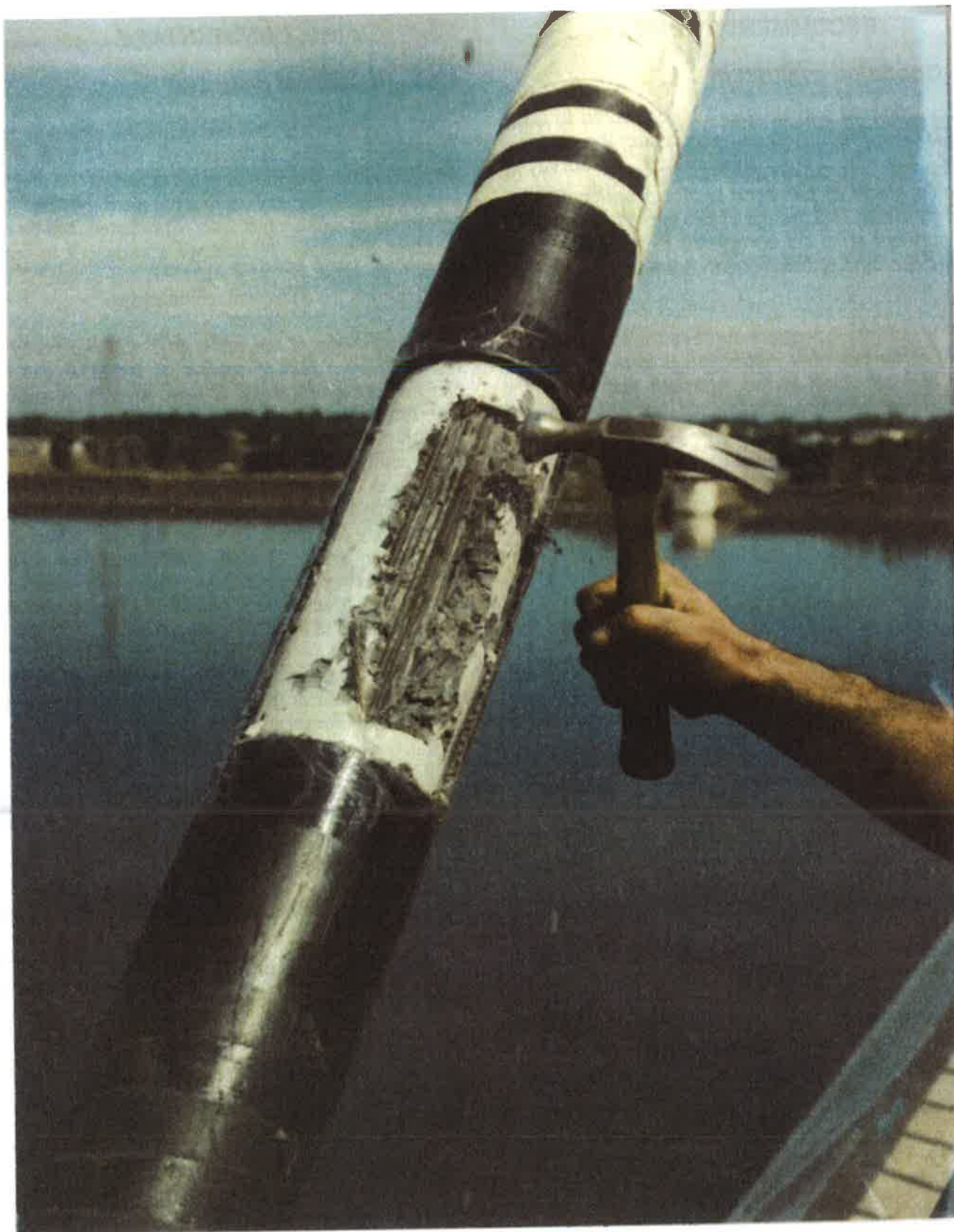
Fig. C7.2—Cable-stay window for Paco-Kennewick Bridge.
